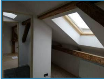
Déva Unitarian Guesthouse room under construction.
